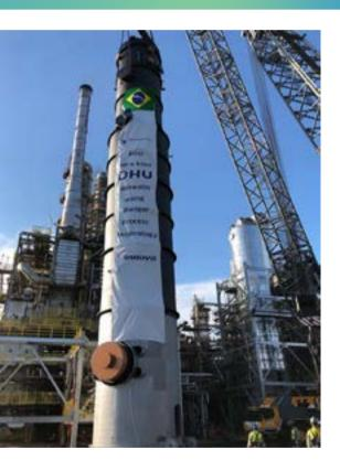
The DHU technology decouples the steam required for the styrene catalyst from heat transfer considerations, which lowers temperatures and facilitates a reduction in steam consumption. Instead of using a fired heater, a simple axial flow heat exchanger with multiple sets of concentric tubes is used, thereby simplifying the styrene unit's complex controls and resulting in easier operations and a safer design.
